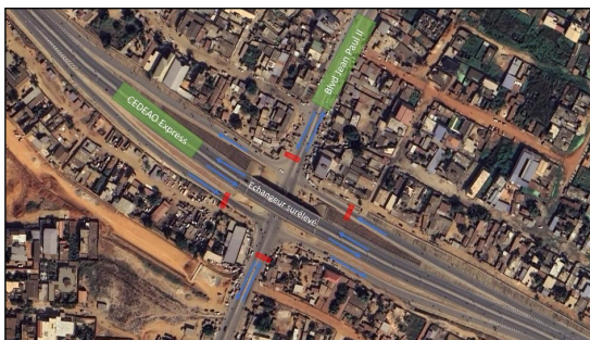
Fig. 6. Overpass of Agoe
