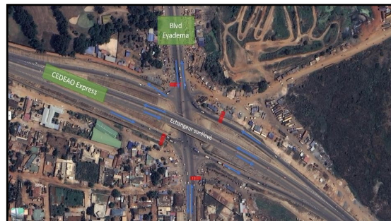
Fig. 7. Overpass of Kegue
