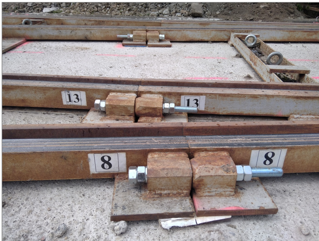
Fig. 8. The numbered segments of overlapping turnouts used during the task of replacing turnouts at the Borek junction
