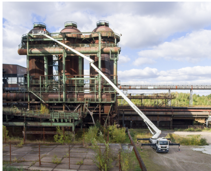
Fig. 2. Mobile platform on a special vehicle [12]
