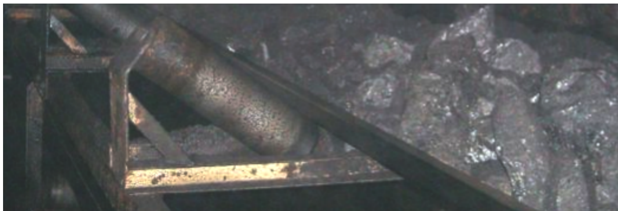
Fig. 1. An example of using a belt conveyor of a coalmine
