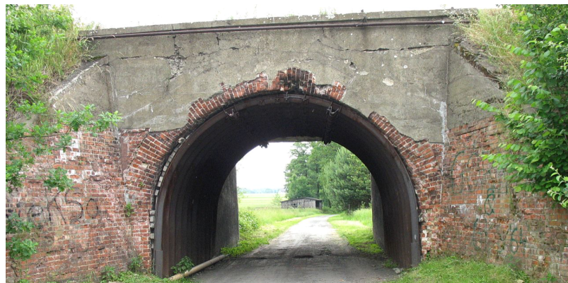
Fig. 3. View of the bridge from the level of the local road
