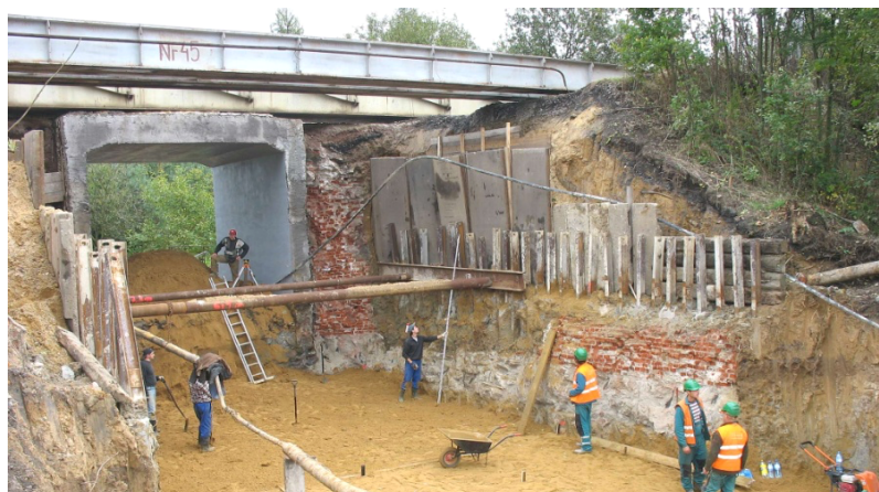
Fig. 2. View of relieving constructions during the rebuilding of the bridge
