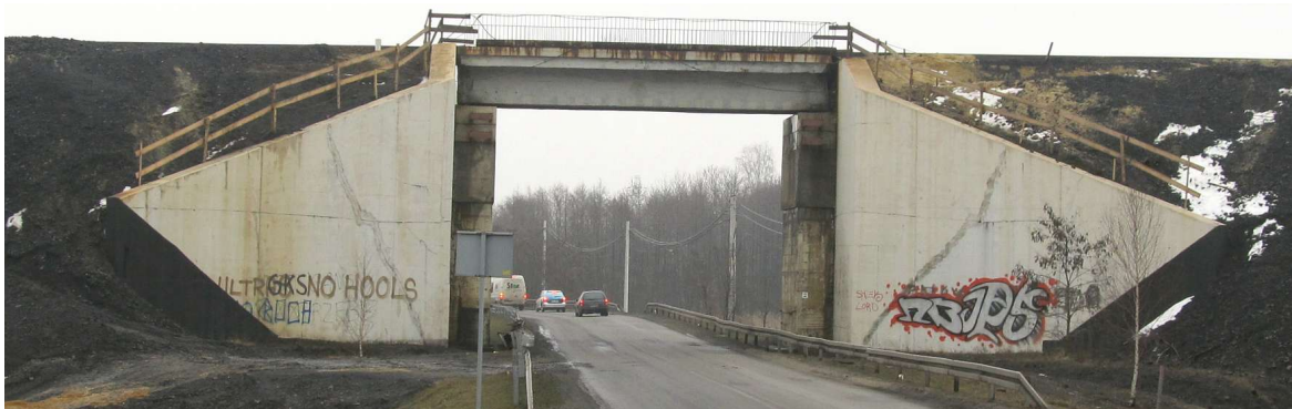
Fig. 7. View of the bridge with the old reinforced concrete span (April 2013)
