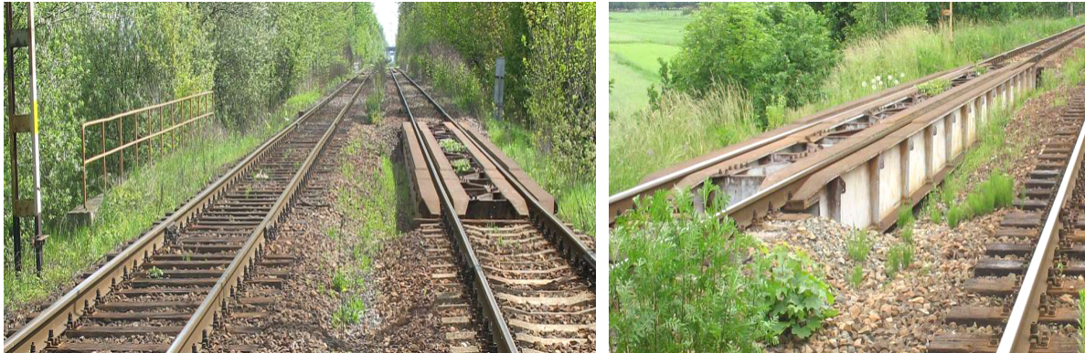
Fig. 5. View of the bridge with a built-in relieving construction
