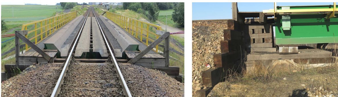
Fig. 10. Relieving construction into the railway, wooden sleepers and temporary wooden back-walls
