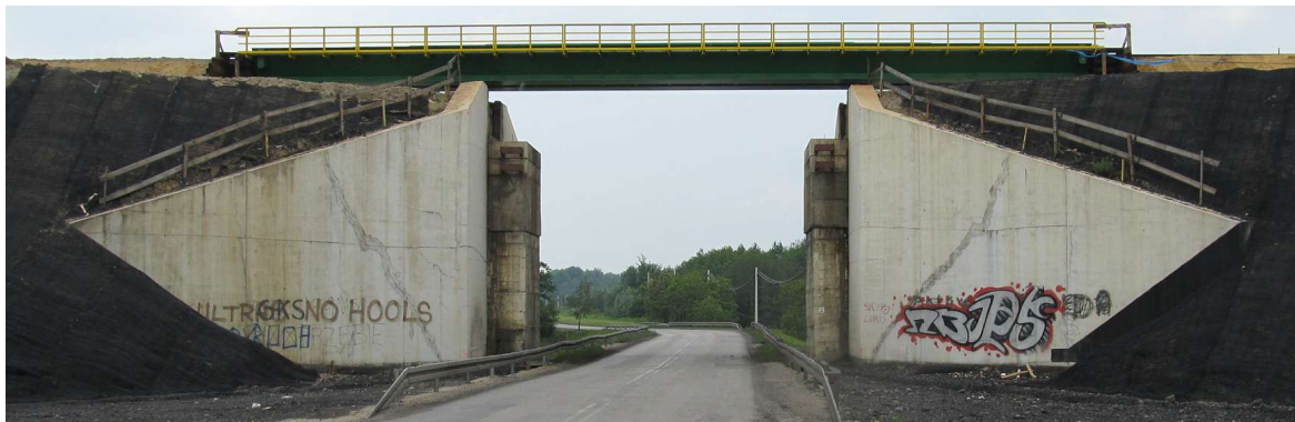
Fig. 8. View of the bridge with steel relieving construction (May 2013)
