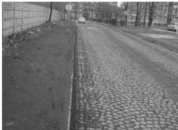
Fig. 7. Cobbled pavement road where measurements were conducted
