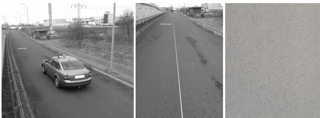
Fig. 2. View of the investigated road section
