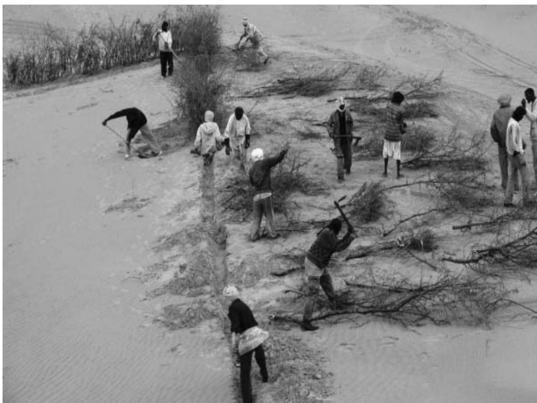
Fig. 1. Ordinary mechanical protection device from materials of vegetable origin
