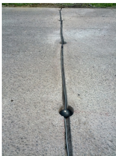
Fig. 3. Installation of temperature sensors in asphalt roads
