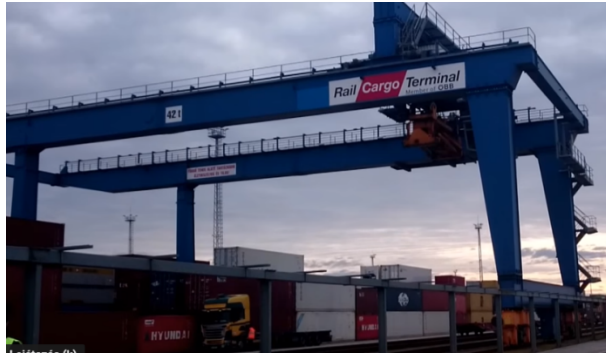
Fig. 1. Gantry crane (source: https://youtu.be/Jcsm3TMT_nM )
