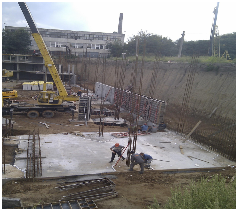
Fig. 2. Erection of the underground parking lot for the residential complex “Panorama”
